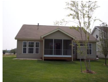
Level Rear Yard
